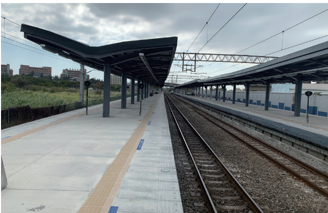
▲ Figure 2-18 Platform alignment work at Peihu Station
